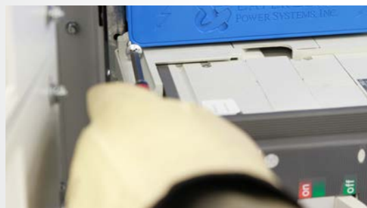
Screws Help Secure The Breaker
