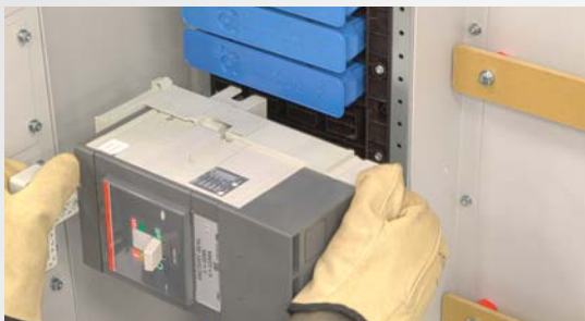
The Breaker Is Inserted Into The SafePanel
